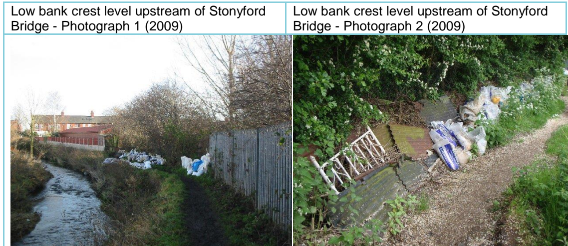
Figure 2-2: Stonyford Bridge photographs
