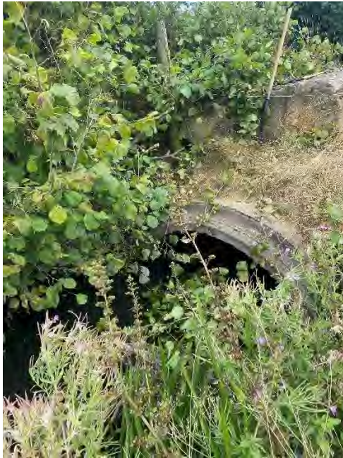
Figure 13. TRIB_007 downstream outlet - 1.75m diameter culvert
