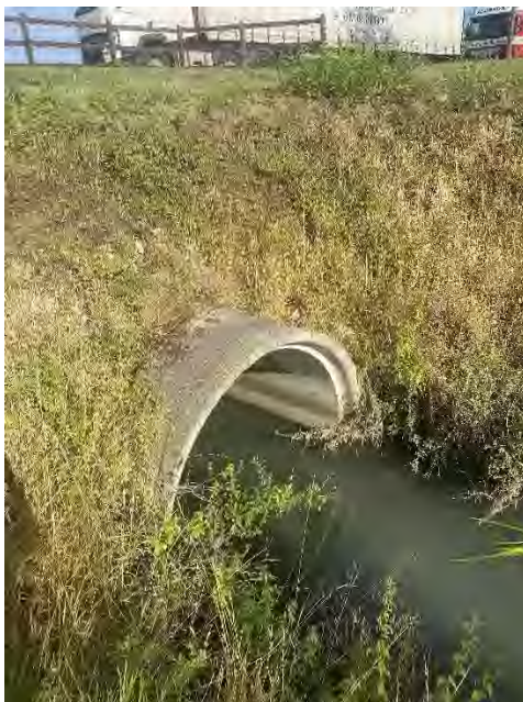
Figure 11. TRIB_002 upstream inlet- 1.9m diameter culvert
