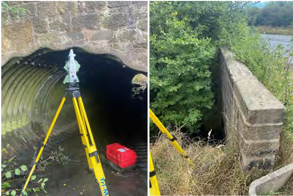
Figure 10. CARR_007 upstream inlet - A635 Culvert
