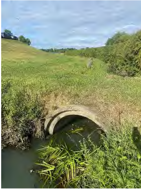
Figure 12. TRIB_004 upstream inlet- 1.35m diameter culvert
