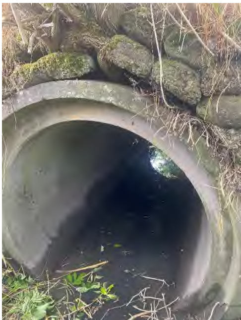
Figure 14. TRIB_011 upstream inlet - 1.5m diameter culvert
