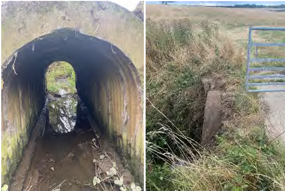
Figure 9. CARR_002 upstream inlet - Farm Access Culvert
