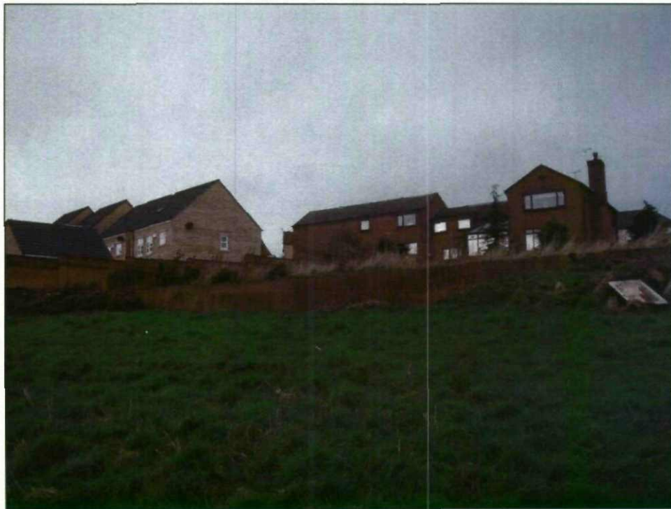
Fig. 12 Modern detached residence in the west of the application area (looking north)
