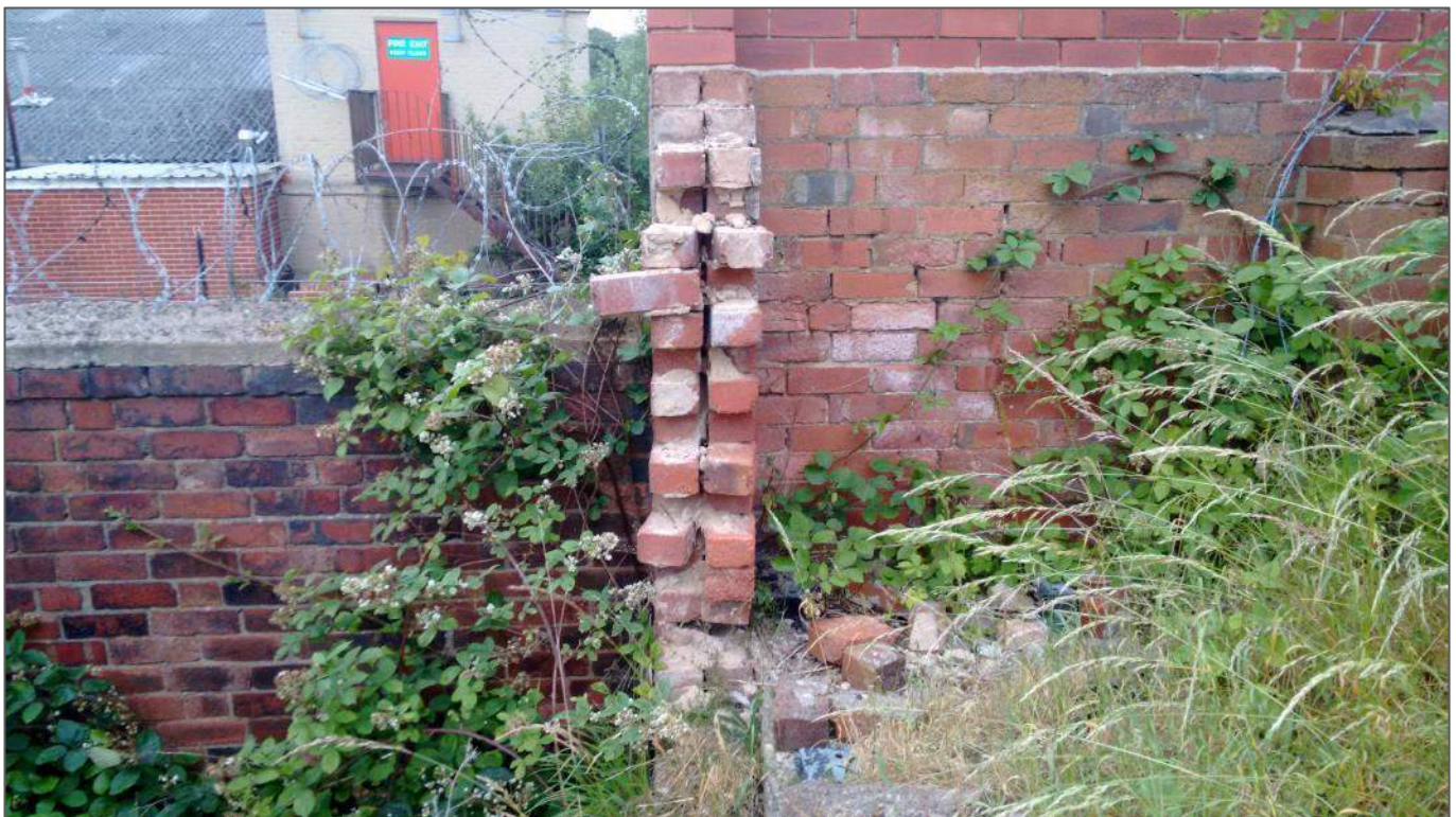
Plate 5: Eastern boundary wall, assessed as having low potential to support roosting bats.
