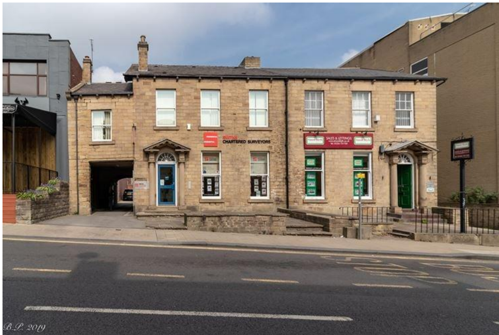
Fig 05. 14 & 16 Regent Street (Grade II listed), visible on the 1850 OS map of Barnsley
