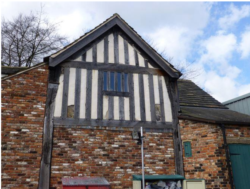
Fig 18. Close-studded gable of 41-43 Church Street
