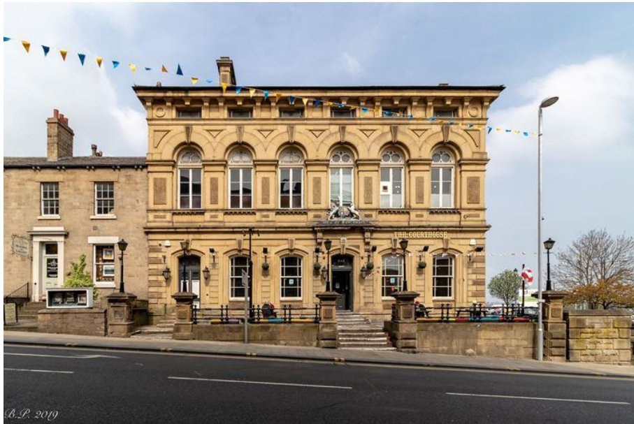
Fig 25. The Courthouse Station (eastern end, north side of Regent Street)
