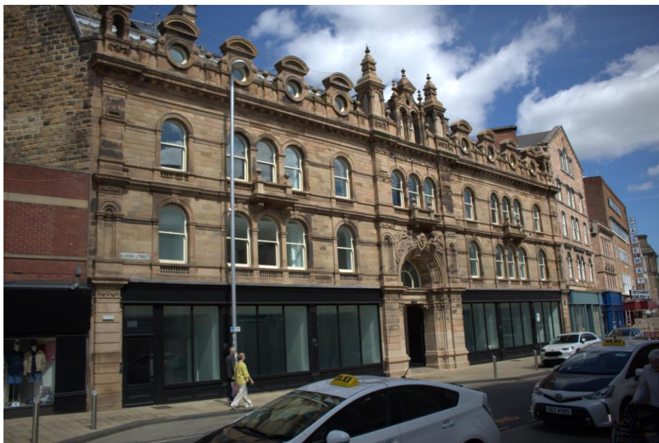
Fig 16. Eldon Street frontage of the Civic Theatre
