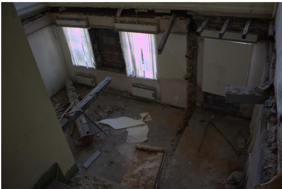
Fig 27. Alterations visible inside 23 Church Street.
