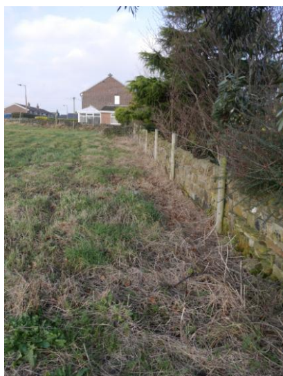
Plate 2: View of the eastern boundary wall, looking north
