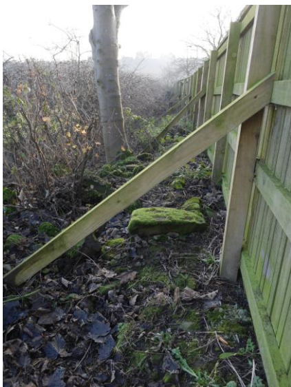
Plate 8: View of the western boundary fence, also showing the remains of the former dry stone wall
