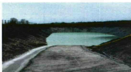
Earth-banked slurry store with access ramp
