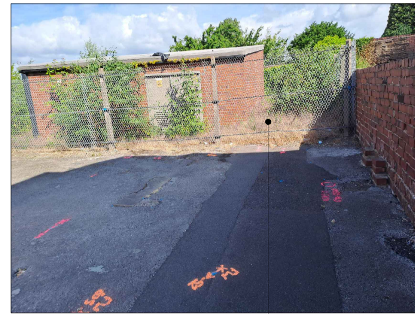
PHOTO 21 Wire mesh fence to NPG Sub-station
