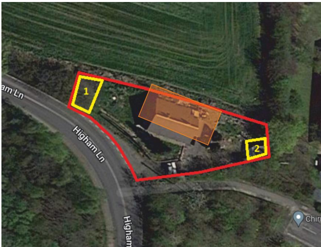
Plate 1: Location of buildings demolished (1 - wooden outbuildings, 2 - detached garages) and approximate position of earlier building (orange)
