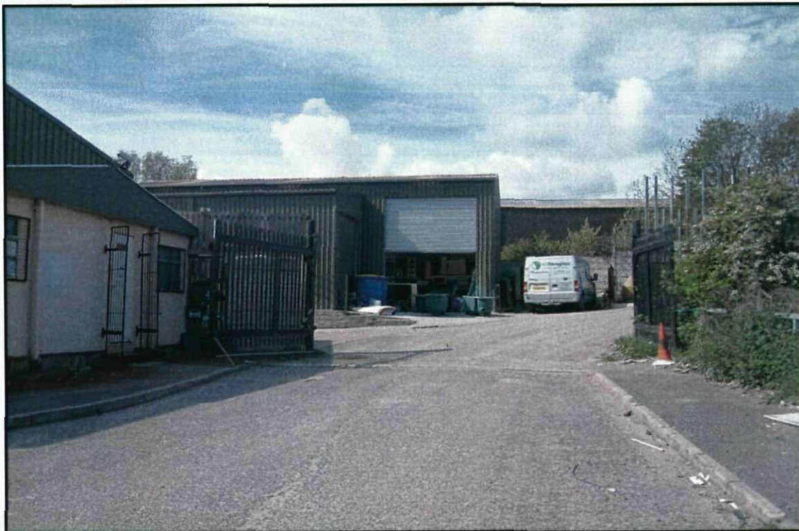
Photograph 4 Entrance to northern yard.
