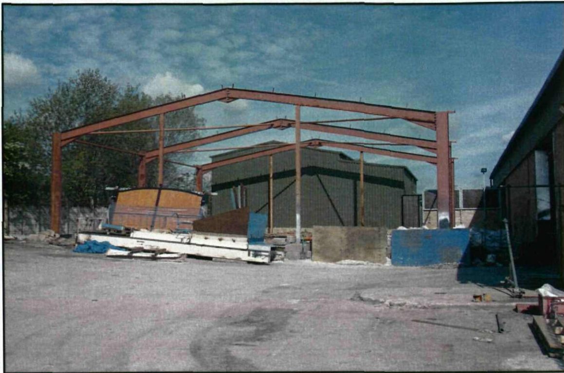
Photograph 3 View showing yard and part constructed portal framed building.
