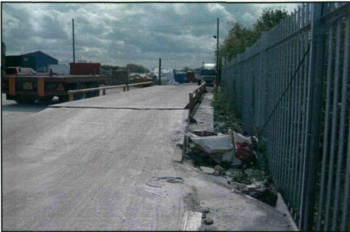
Photograph 9 View of weighbridge along south-western boundary.
