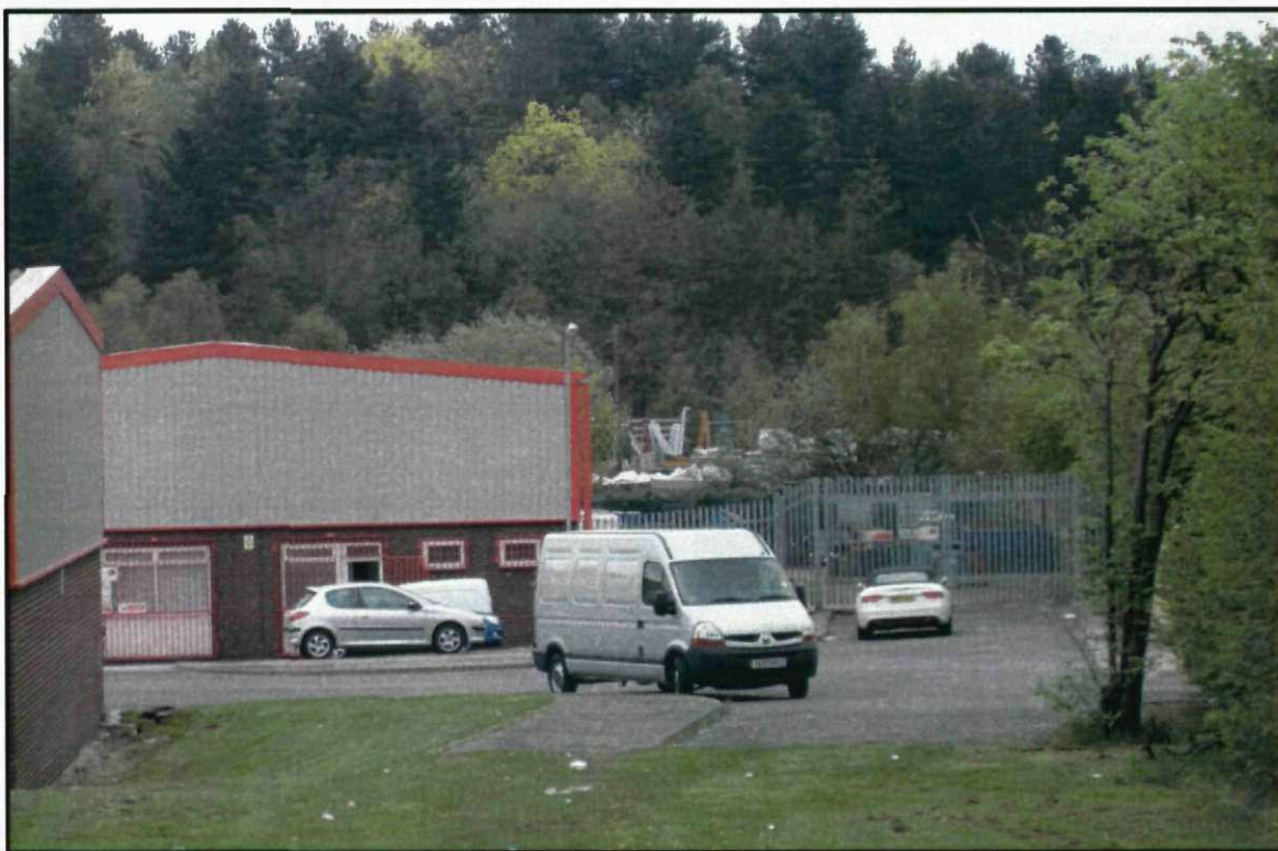
Photograph 14 Industrial premises to south-west of site, partially on infilled canal.
