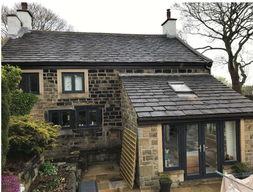
Fig 06. Rear (West) Elevation to White House Farm.
