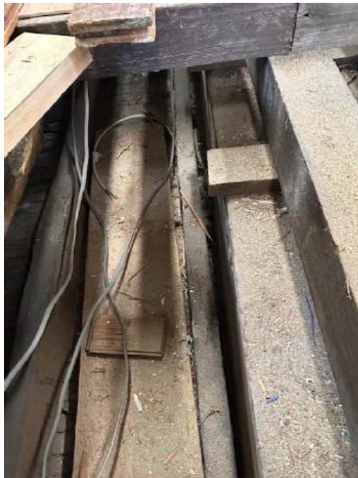
Figure 121. Timber board seen resting on plaster laths and nibs.
