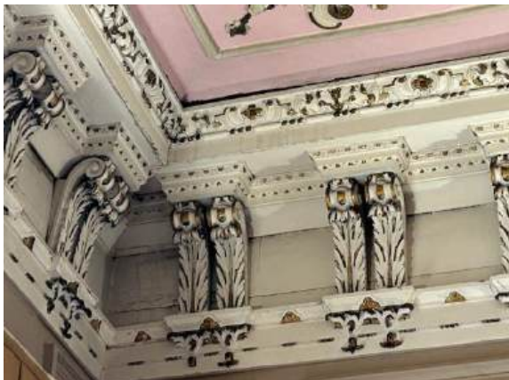
Figure 41. Splitting and ingress observed on the South wall cornice and ceiling.
