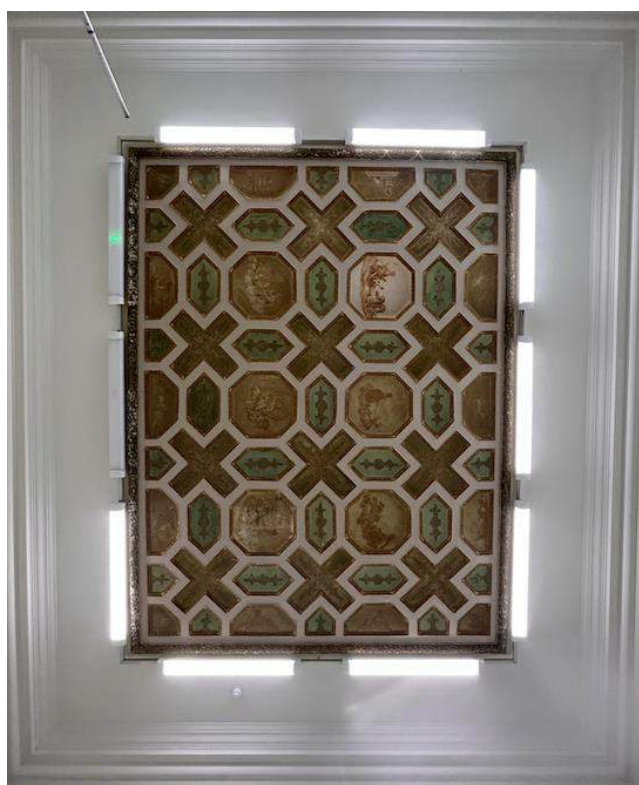
Figure 87. I.C.T. Teaching Room 1 Plaster Ceiling.
