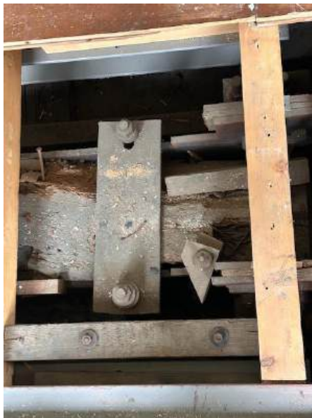
Figure 13. Bolts visible from the upper side of the ceiling matching the location of the bolts visible on the underside of the ceiling.
