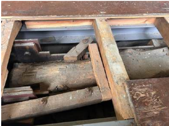
Figure 19. Earlier steels shown supporting timber beam with grey coated beams inserted parallel to the timber beams.
