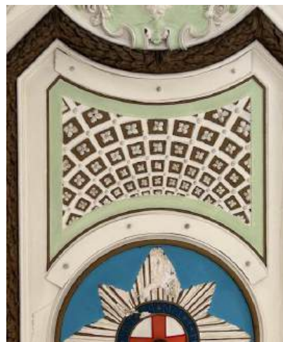
Figure 50. Support straps attached with bolts.
