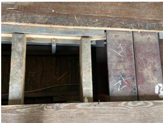
Figure 17. Red coloured steel beams running East to West give evidence of the first major intervention to the ceiling's structural stability.
