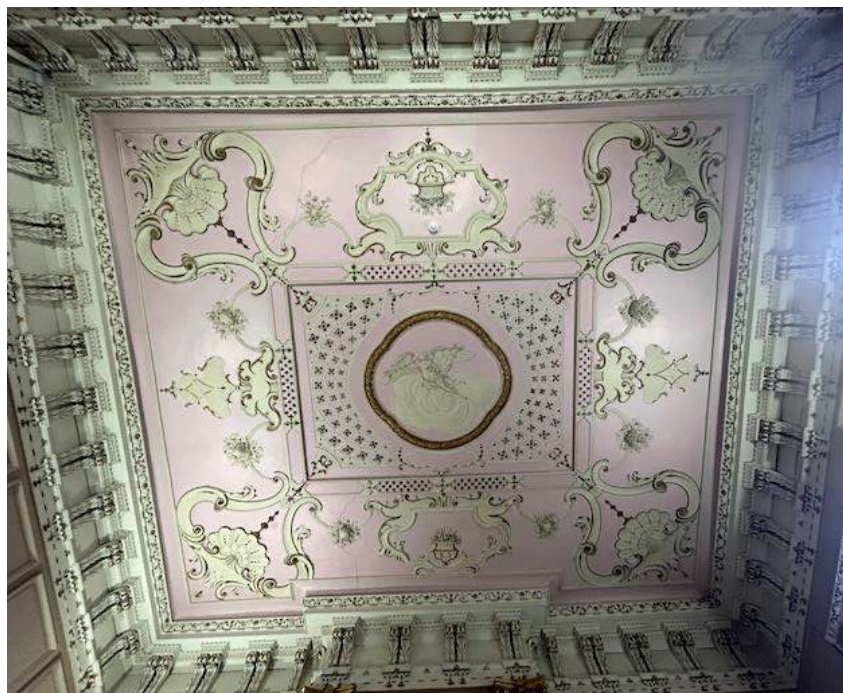
Figure 38. Queen Anne Suite 3 Ceiling.
