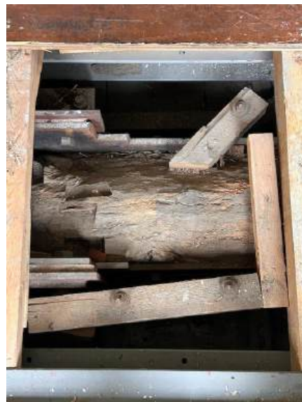
Figure 24. Loose timber elements affixed with bolts requiring extra stabilization agreed upon with architect.
