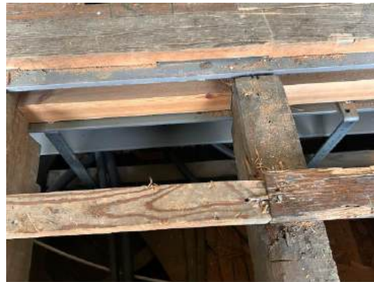
Figure 22. Steel beams found where timber beam would have originally been.
