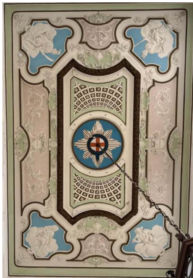
Figure 46. Italian Staircase Plaster Ceiling
