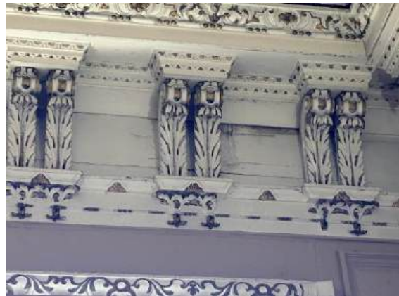
Figure 40. Splitting and ingress visible on the East wall cornice.
