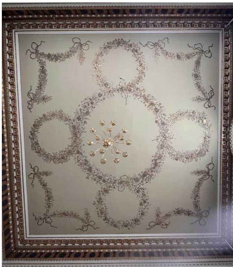
Figure 112. Principal's Office Ceiling.
