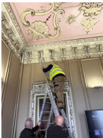
Figure 43. A loose embellishment was removed above the West wall during the survey due to being a hazard to visitors to the room.
