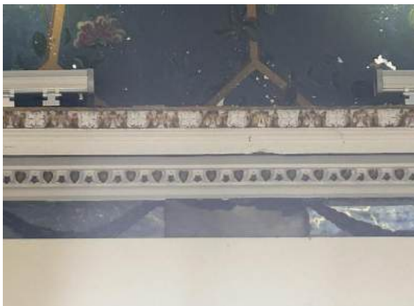
Figure 107. Loss of mirrored frieze panel.
