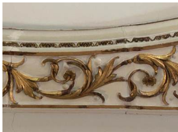
Figure 11. Bolts visible give evidence on the underside ceiling of the stabilization methods which occurred on the upper side of the ceiling.
