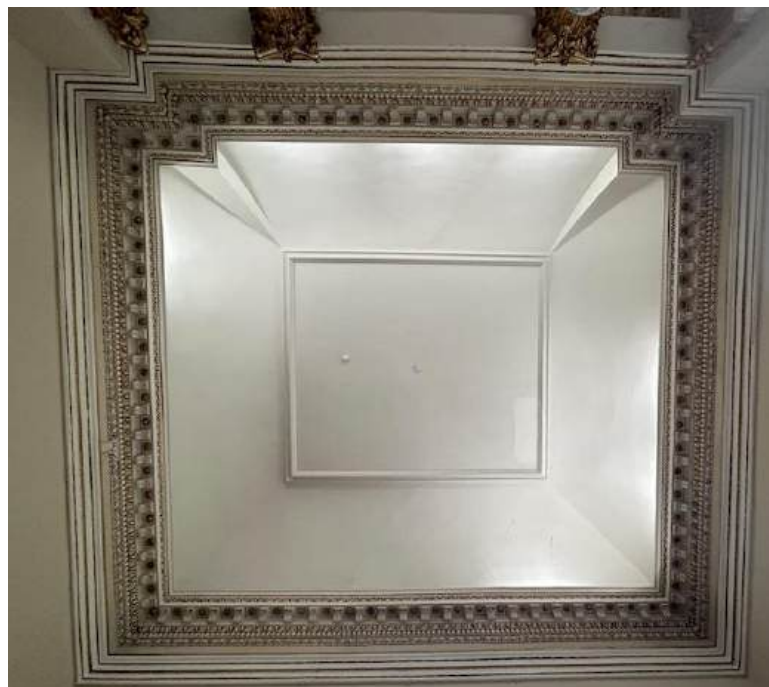
Figure 52. Long Gallery North End Room Plaster Ceiling.
