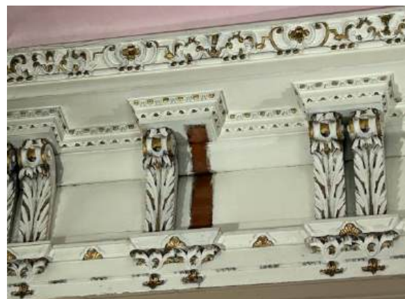
Figure 44. Removed loose embellishment revealing the cornice to be made of timber.
