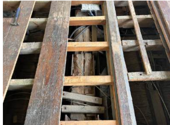
Figure 20. Timber beam supported by steels on either side.
