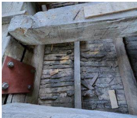
Tight lath and minimal key, previous interventions visible.
