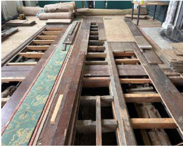
Figure 15. Access to upper side of the ceiling was provided by expanses of the floorboards being lifted.
