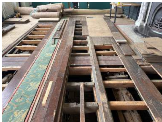
Figure 23. Two red steel beams inserted East to West above timber beams.
