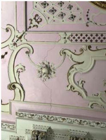
Figure 39. Hairline cracks visible throughout the ceiling and cornice.
