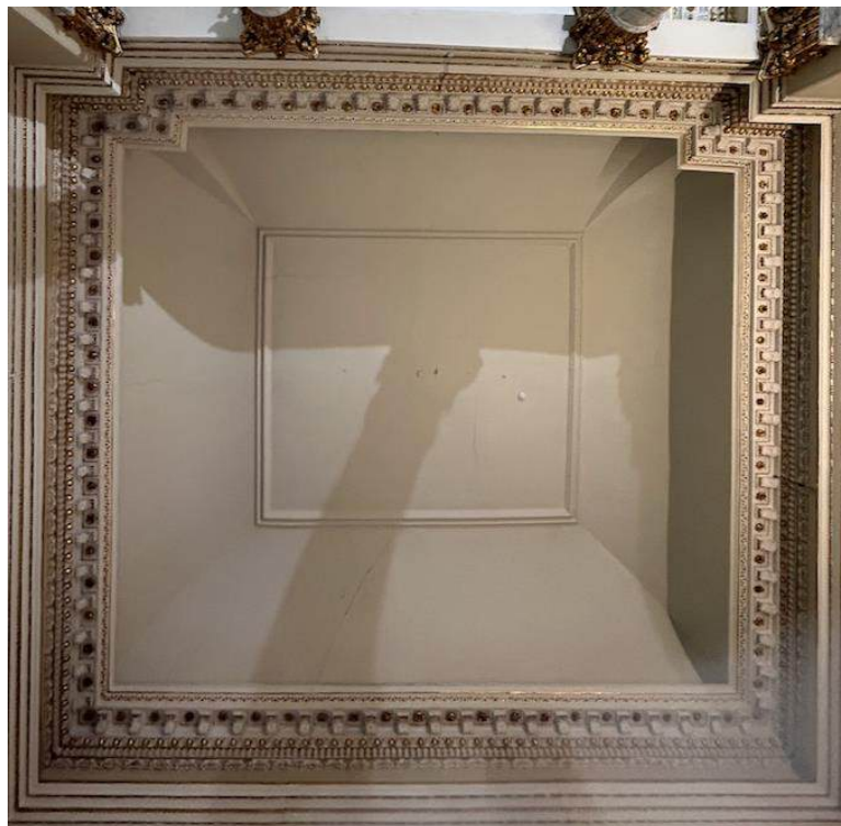
Figure 68. Long Gallery South End Room Plaster Ceiling.
