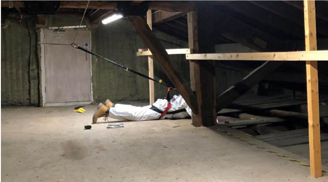
Figure 71. Keith Langton inspecting the topside of the ceiling, note location of hoist and boarded floor, limiting access for inspection. Shown at *4 in the diagram below.
