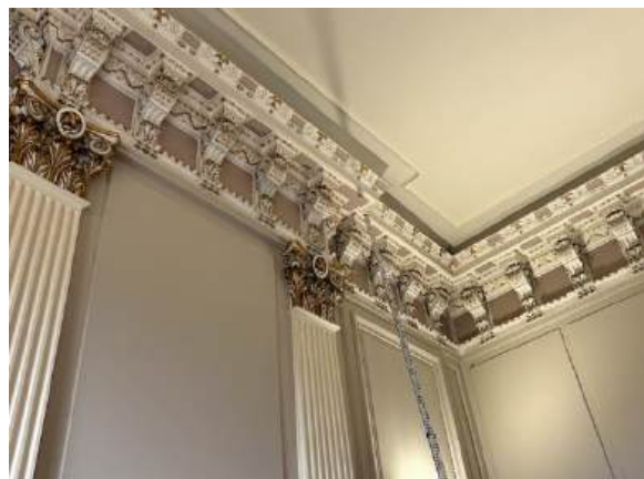
Figure 30. Push test revealed the plaster ceiling to be stable.
