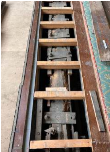
Figure 21. Timber beams being aided by later added support system.
