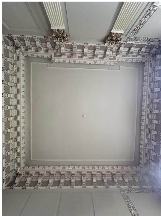
Figure 26. Queen Anne Room 1 Plaster Ceiling.
