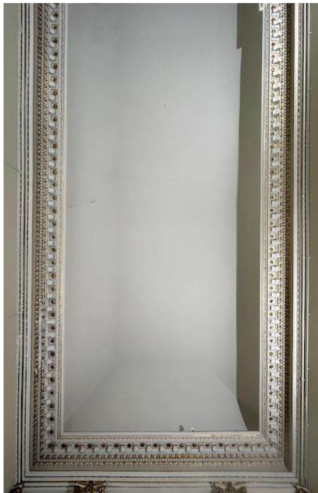
Figure 64. Long Gallery South Section Ceiling.
