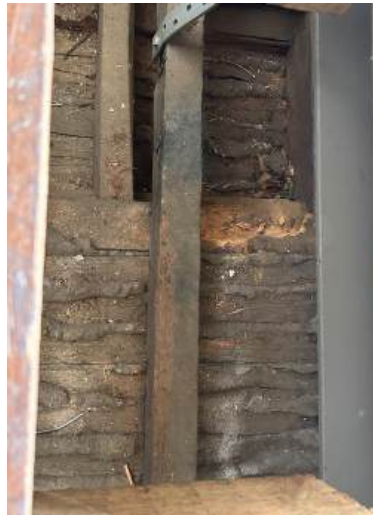
Figure 17. Close up of ribs and laths.
