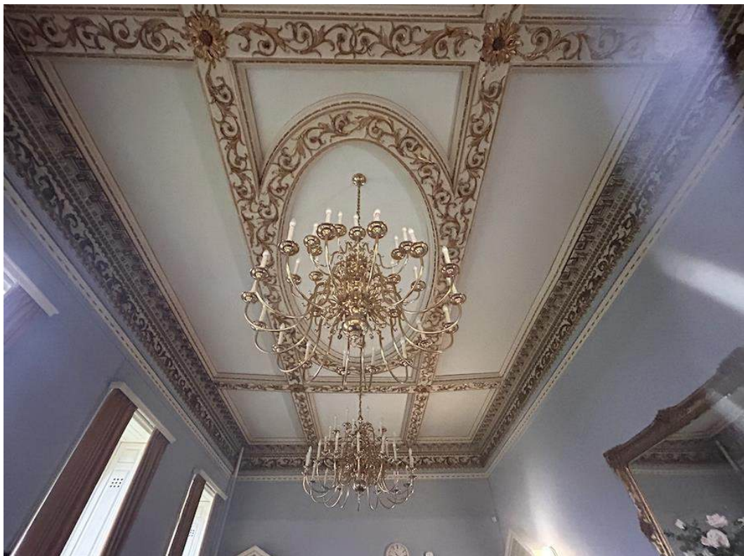
Figure 5. Blue Room Decorative Plaster Ceiling.
