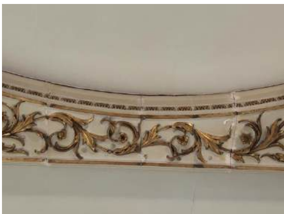
Figure 10. Equally spaced fractures which could be deliberate cuts from upper ceiling stabilization work.
