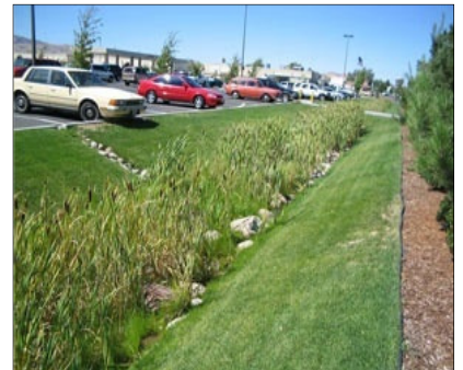
Figure 6-5: Indicative one way cross fall design (left) and constructed vegetated swale (right)
