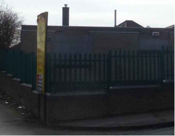
Existing boundary wall (A) to be retained and replicated as wall (B). Palisade fence to be removed.
