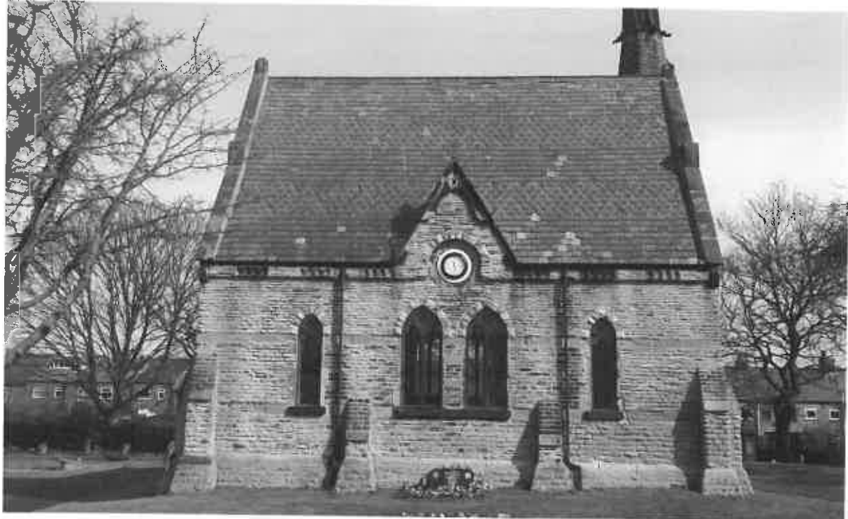
Side Elevation of the North chapel
