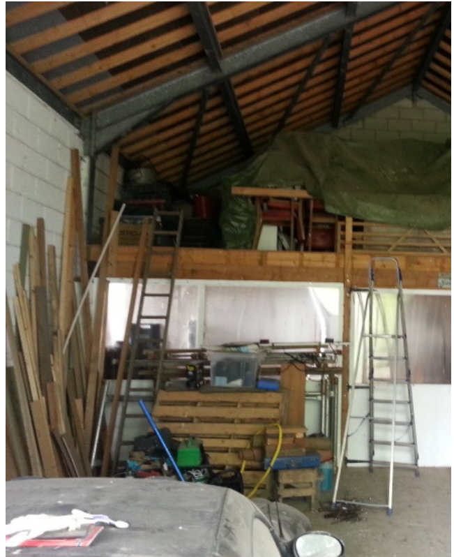
Figure 8 – (Top) The West elevation from the south Figure 9 – (Middle) The East elevation from the south Figure 10 – Internal view showing mezzanine storage
