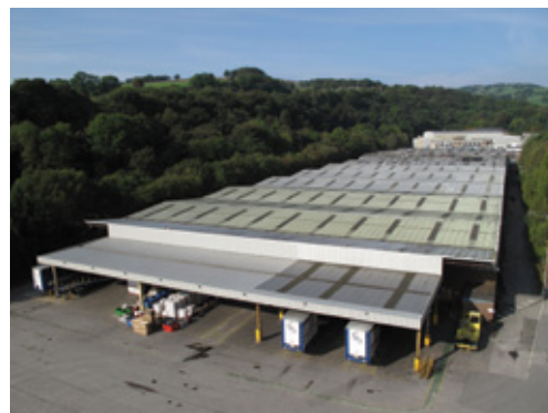
AERIAL OF BUILDING B21 WAREHOUSE WITH CANOPY
