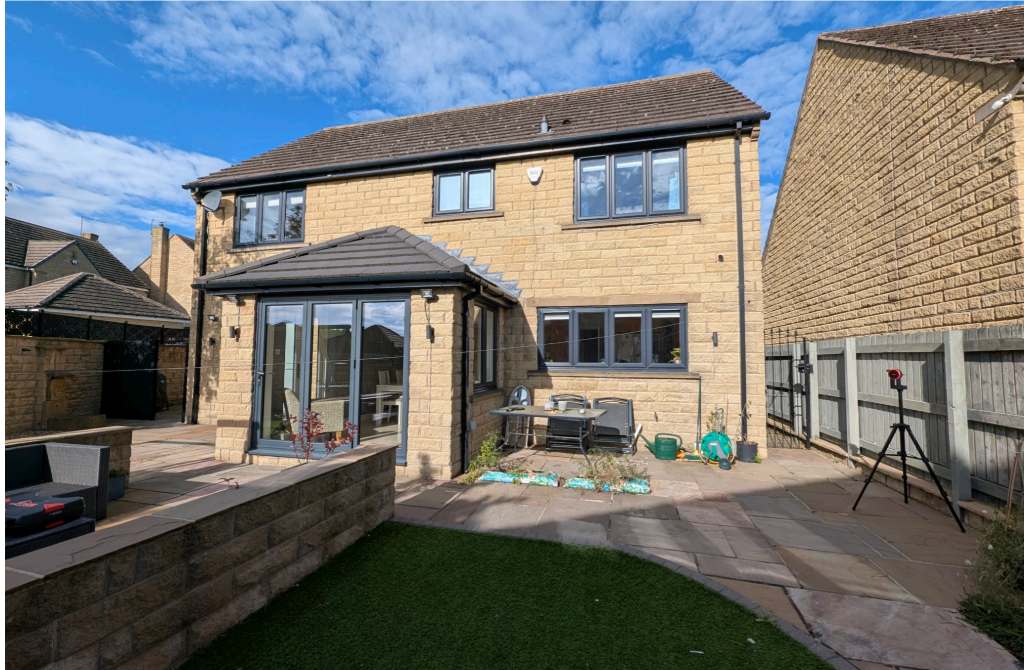
2507 - 2 Brookfields, Oxspring, S36 8WG Existing SE (rear) Elevation
