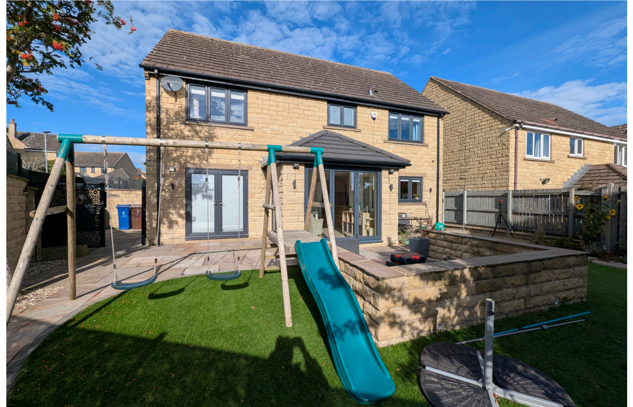
2507 - 2 Brookfields, Oxspring, S36 8WG Existing SE (rear) Elevation
