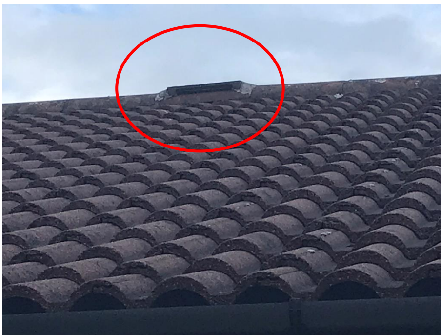
Photograph 13 – Vent providing access to a possible loft void ( TN8; Figure 1 ). One instance. Photograph taken of B3 .
