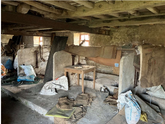
Fig 03. Milking parlour and first floor steel and timber beams supporting stone flags.
