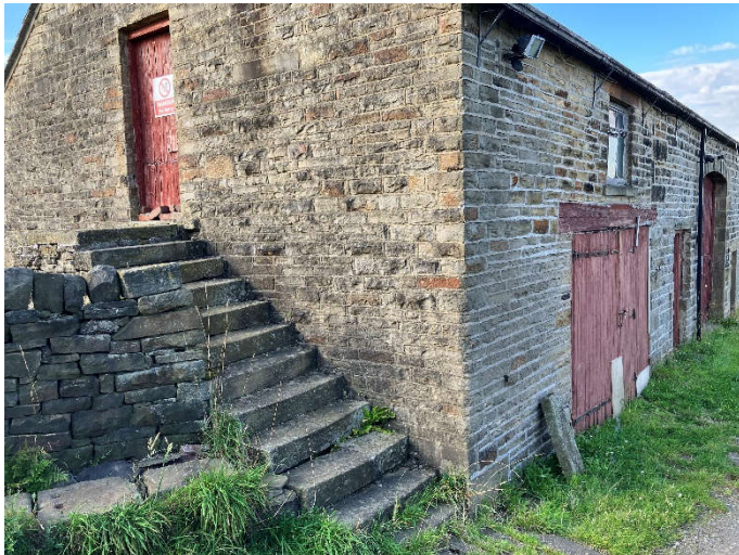
Fig 06. Stone steps and access to first floor hay loft in west gable.
