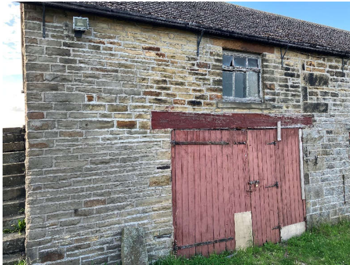
Fig 05. Small addition to west of main barn; note straight joint to reveal of door opening. Construction techniques suggest it was erected soon after completion of the main barn.
