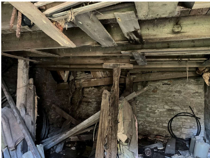
Fig 07. Partial collapse of timber first floor and temporary support posts.
