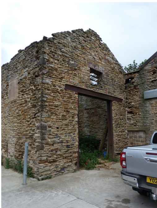
2. South west gable
