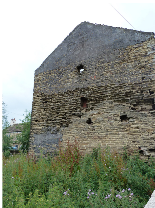
3. North east gable
