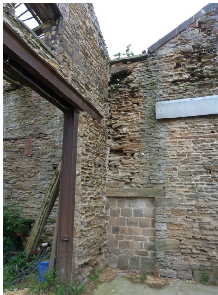
8. Large opening to south gable
