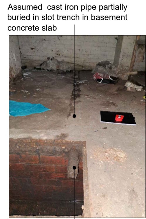
Approx 3" cast iron pipe entering sump chamber at high level
