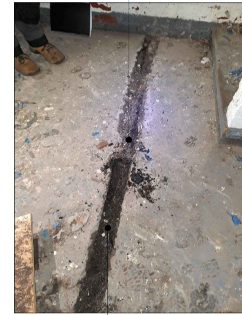
Potential drainage channel in concrete slab of cellar of No.305 (thought to feed into sump chamber of No.303 cellar)
