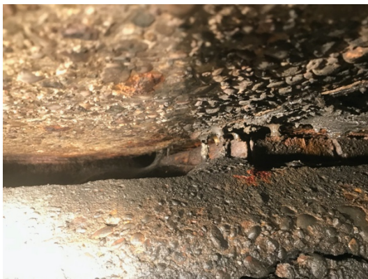
Image 3: Cobwebs in cavities of bridge
