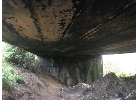
Image 2: Underside of bridge deck
