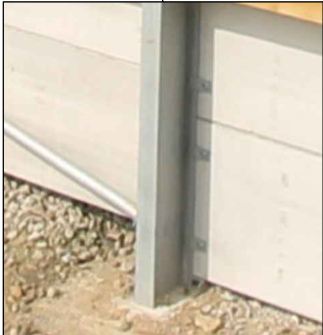
Galvanised Columns & Steelwork and Concrete Panels
