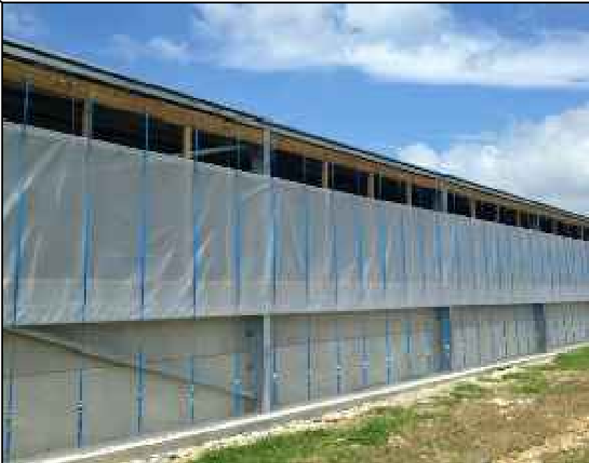
Automated rise and fall curtains full length of the building to the North & South elevations
