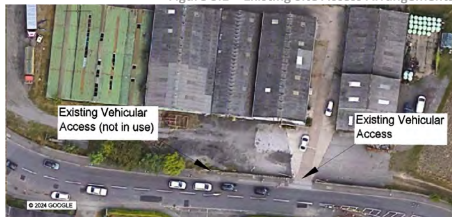
Figure 3.1 – Existing Site Access Arrangements
