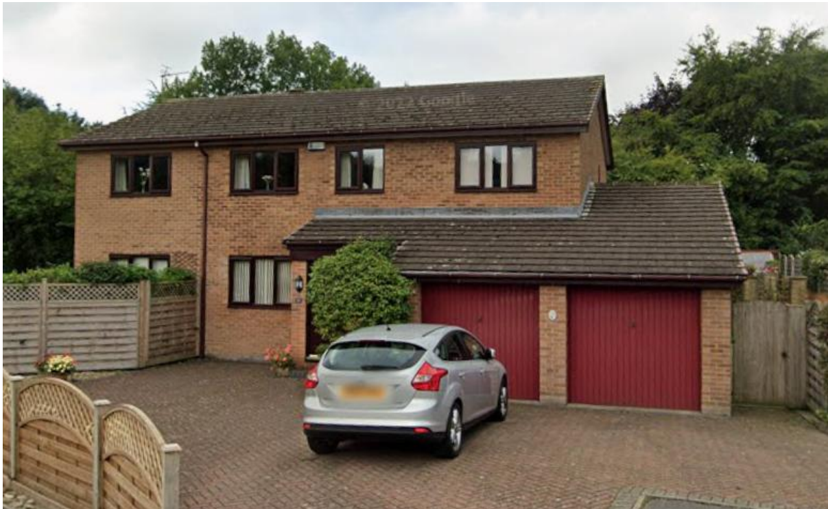
Existing two storey side extension at no.22 Windermere Road, facing the SW elevation of the application site.
