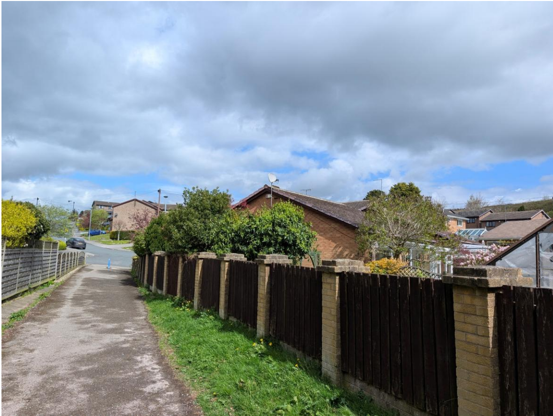
Existing Side & Rear Elevation from Water Hall Park access footpath
