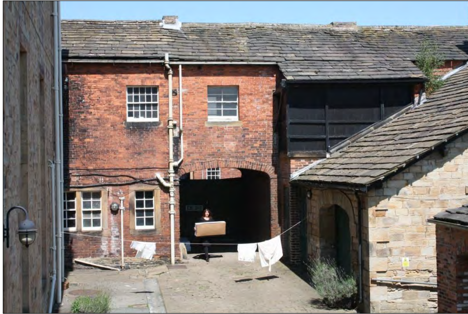
COTTAGE NO 1 – REAR ELEVATION FACING SOUTH
