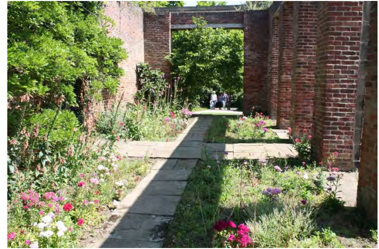
INTERNAL PAVED GARDEN IN POOR REPAIR
