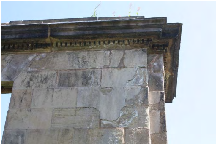
CEMENT FACING AND POINTING TO END WALLS
