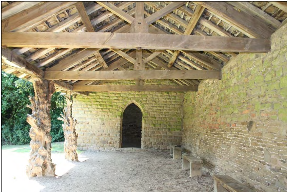
INTERNAL TIMBER STRUCTURE
