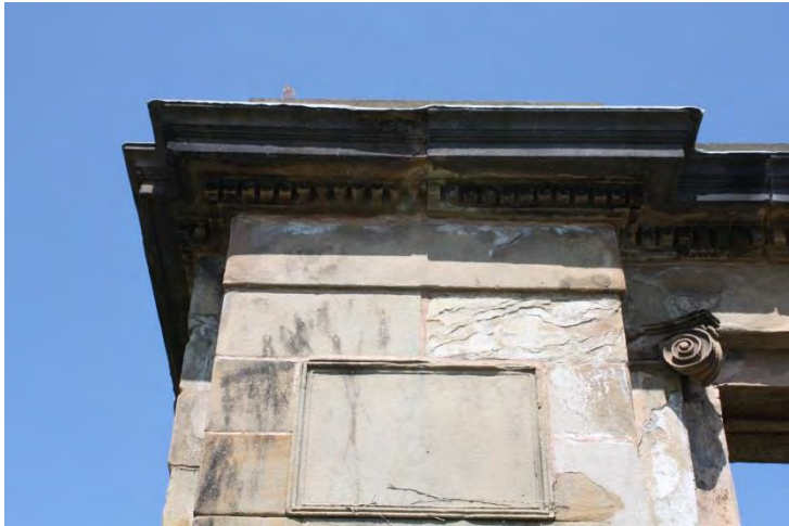
DISPLACE CORNICE TO WEST CORNER PIER
