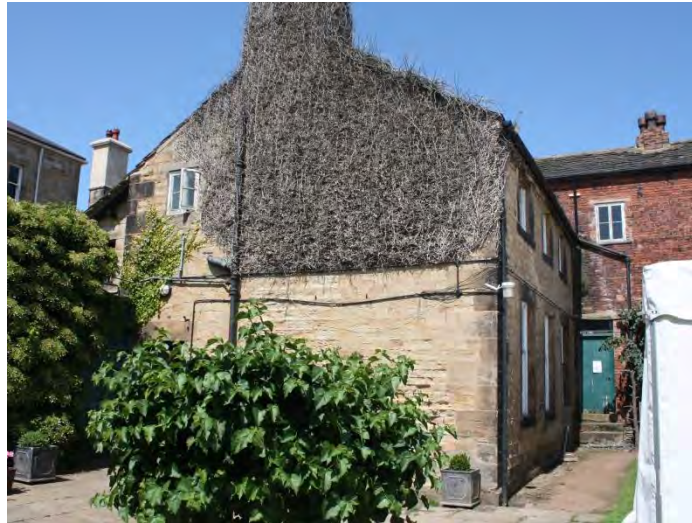
SOUTH FACING ELEVATION
