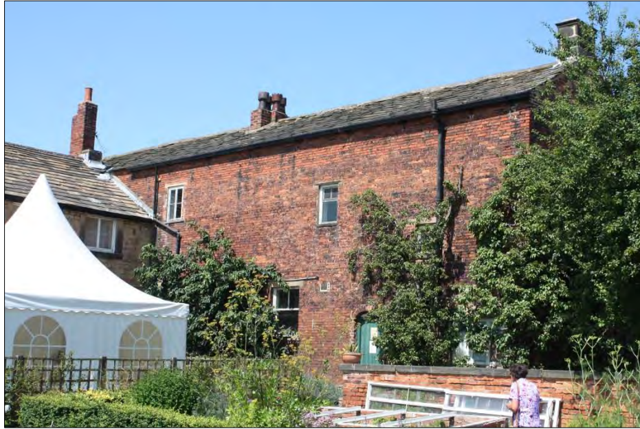
COTTAGE NO 2 – REAR ELEVATION FACING SOUTH
