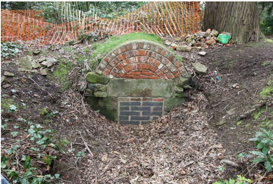
PARTIALLY BURIED ENTRANCE TO THE ICE HOUSE
