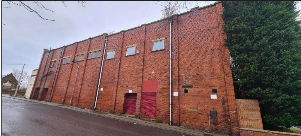
Plate 4. The cinema viewed from the road to the southeast of the site
