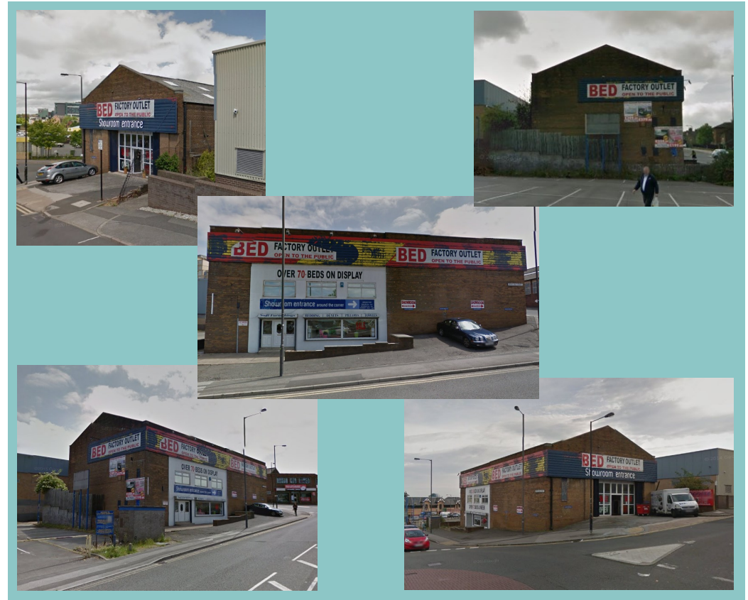
Images of the Existing Building
