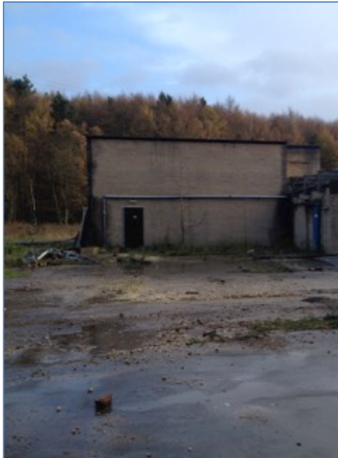
Photograph 1. Hard-standing south of building B4, with woodland beyond
