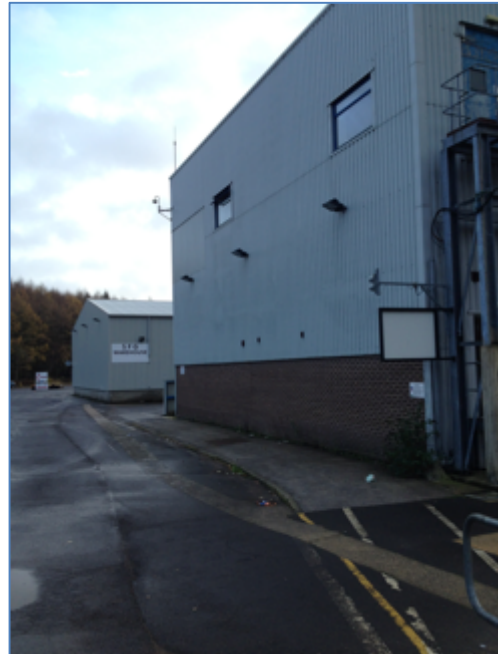
Photograph 2. Hard-standing in front of building B19, viewed from the bridge
