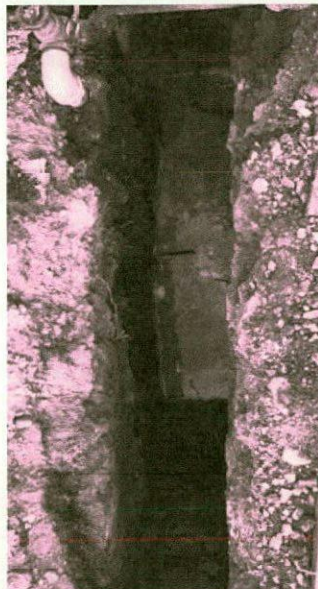
Plot 6: Approx. 0.40m made ground over what appears to be clayey gravelly sand.
