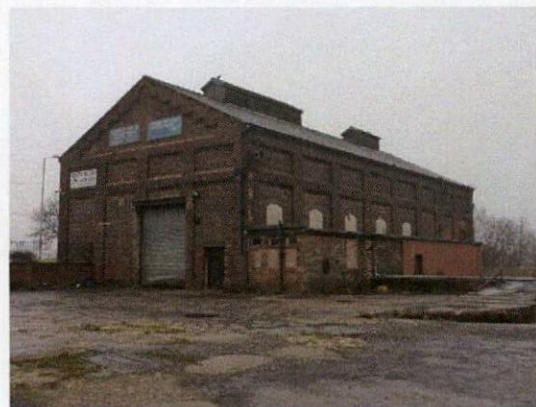
View of existing building on site
