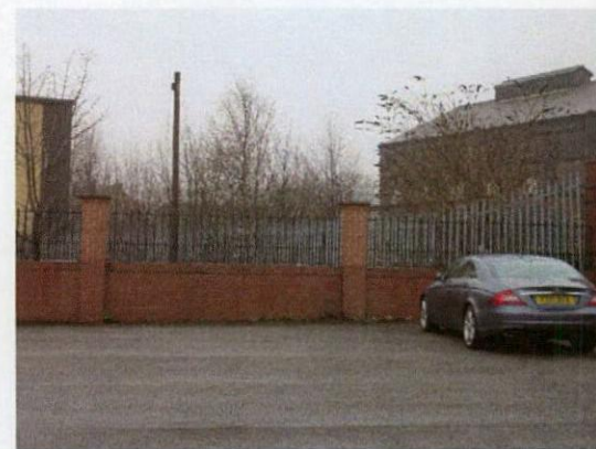
View of wall to boundary with Rockingham business park
