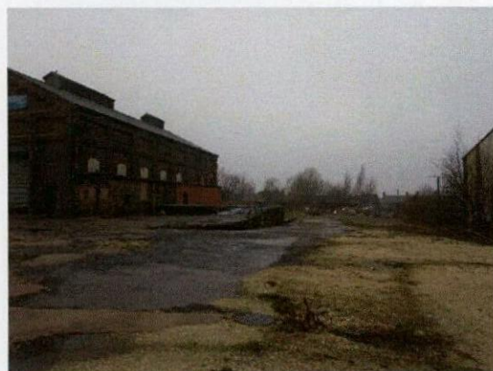
View across site looking North
