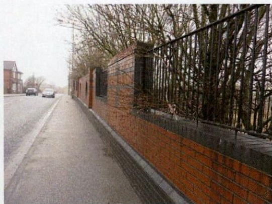
View along boundary wall to Sheffield Road
