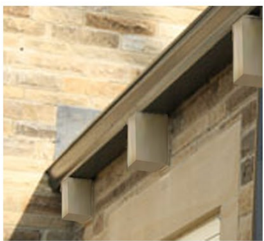
6 GRP Artstone effect band underneath GRP Artstone effect corbels
