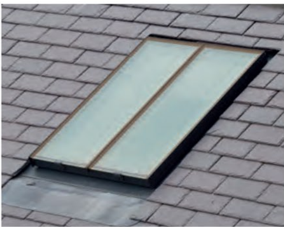
Natural slate adjacent Conservation Rooflight 1 Natural slate on outside faces only and flat roof membrane in dark grey to internal faces
