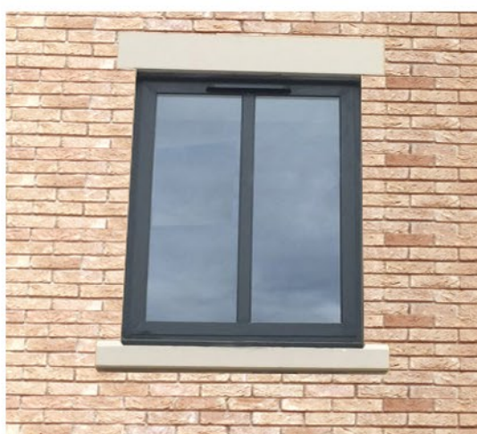
7 Upvc windows - Colour: anthracite with Art. stone cill and head
