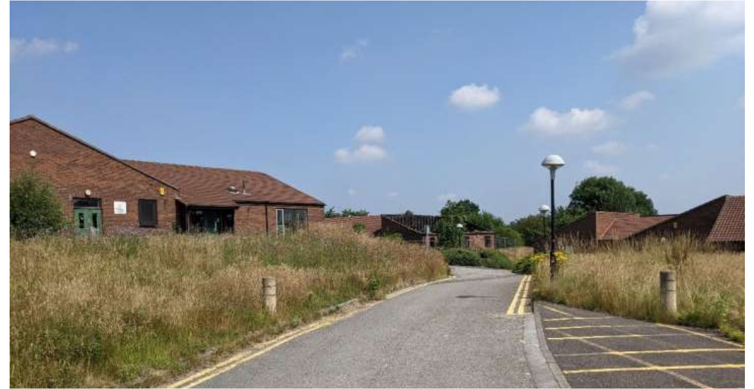
DISUSED NHS BUILDINGS
