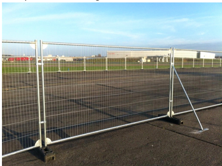
Tree protection fencing
