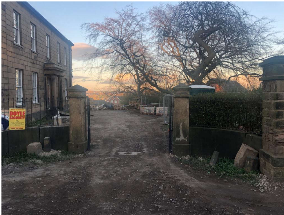
Fig 02. View of existing entrance with stone gate posts set within semi-circular ashlar low wall to entrance area and stone piers to outer corners.
