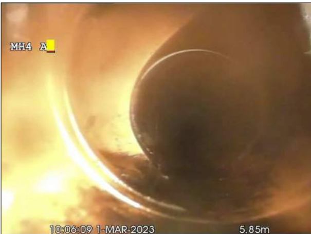
Photo: 33_6a, 00:00:00 5.85m, Junction at 09 o'clock, dia 100 mm
