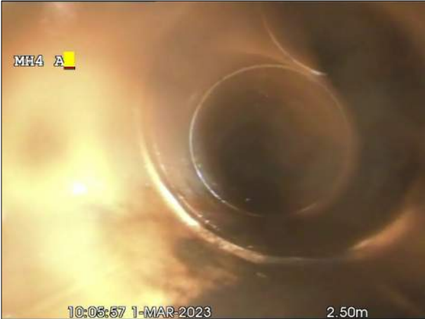
Photo: 31_4a, 00:00:00 2.5m, Junction at 12 o'clock, dia 100 mm
