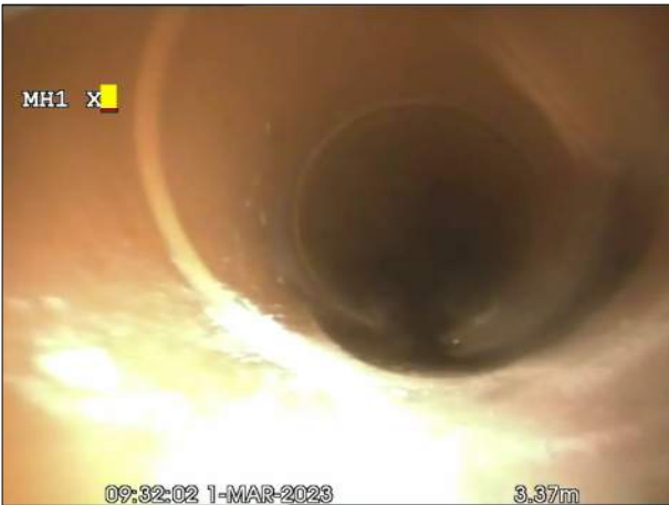
Photo: 12_4a, 00:00:00 3.4m, Junction at 02 o'clock, dia 100 mm
