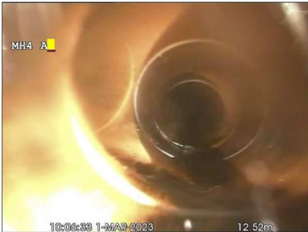
Photo: 35_8a, 00:00:00 12.5m, Junction at 09 o'clock, dia 100 mm
