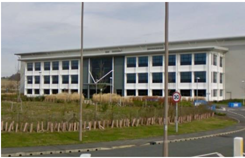
Fig. 5 ASOS office opposite site
