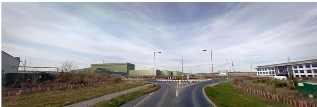
Fig. 43 Eye level view of proposed facility from northbound A6195 Park Spring Road
