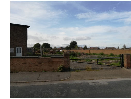
Access from Blackheath Road
