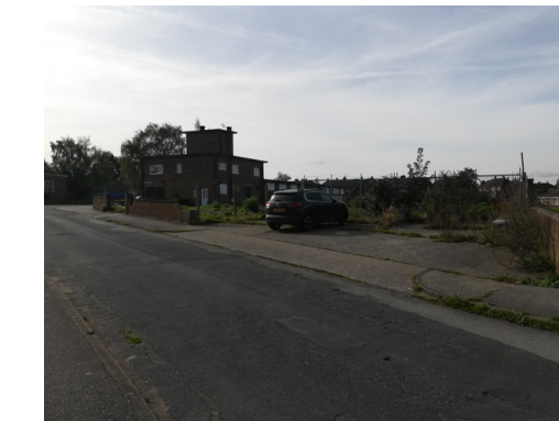
Access from Blackheath Road
