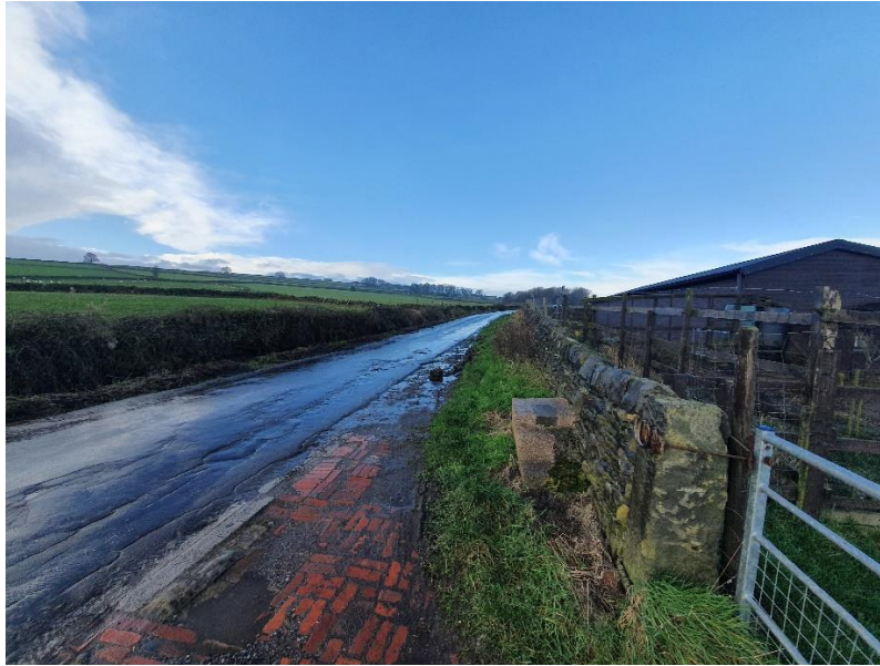
Photograph 3: Site frontage (westbound)
