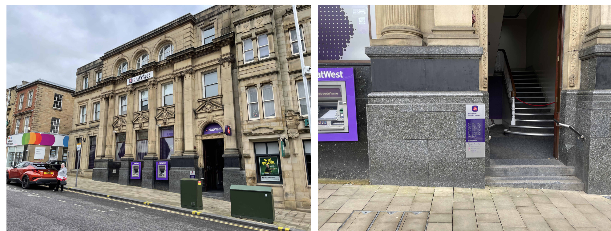
1. Main View of Market Hill Rd
