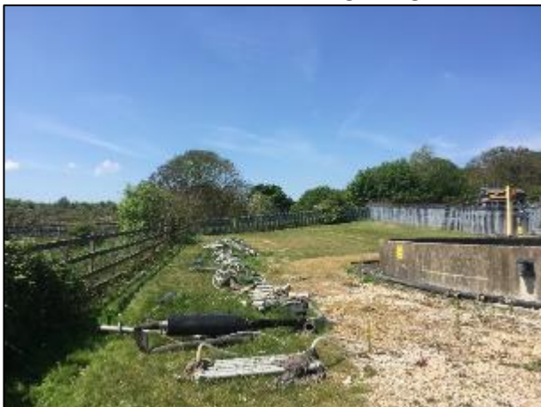
Photograph 17: Examples of TN4; pipes and other debris in current works becoming overgrown
