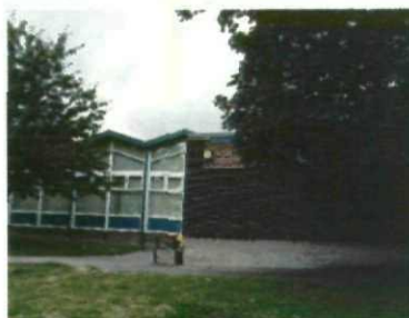
Photograph B – Pitched and flat sections
