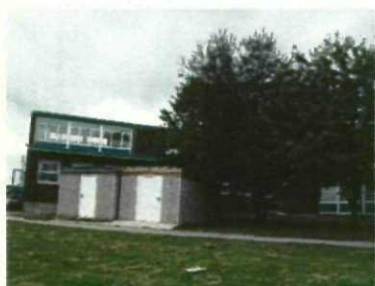
Photograph A – Flat roof section
