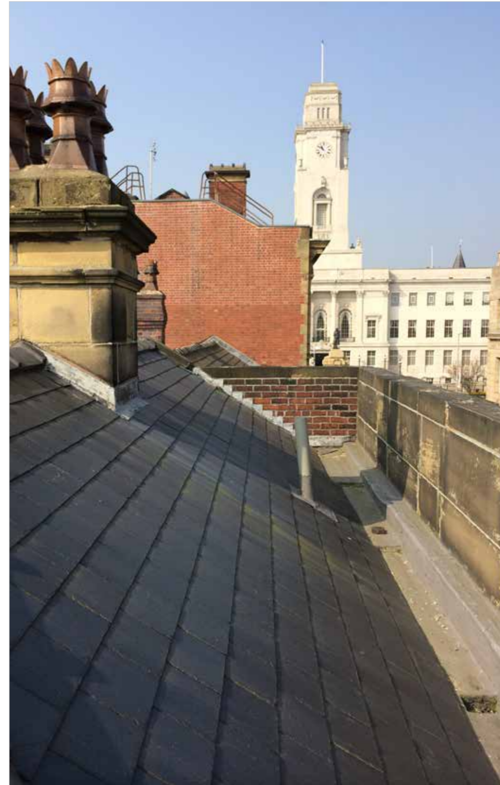
Existing Roof Looking West
