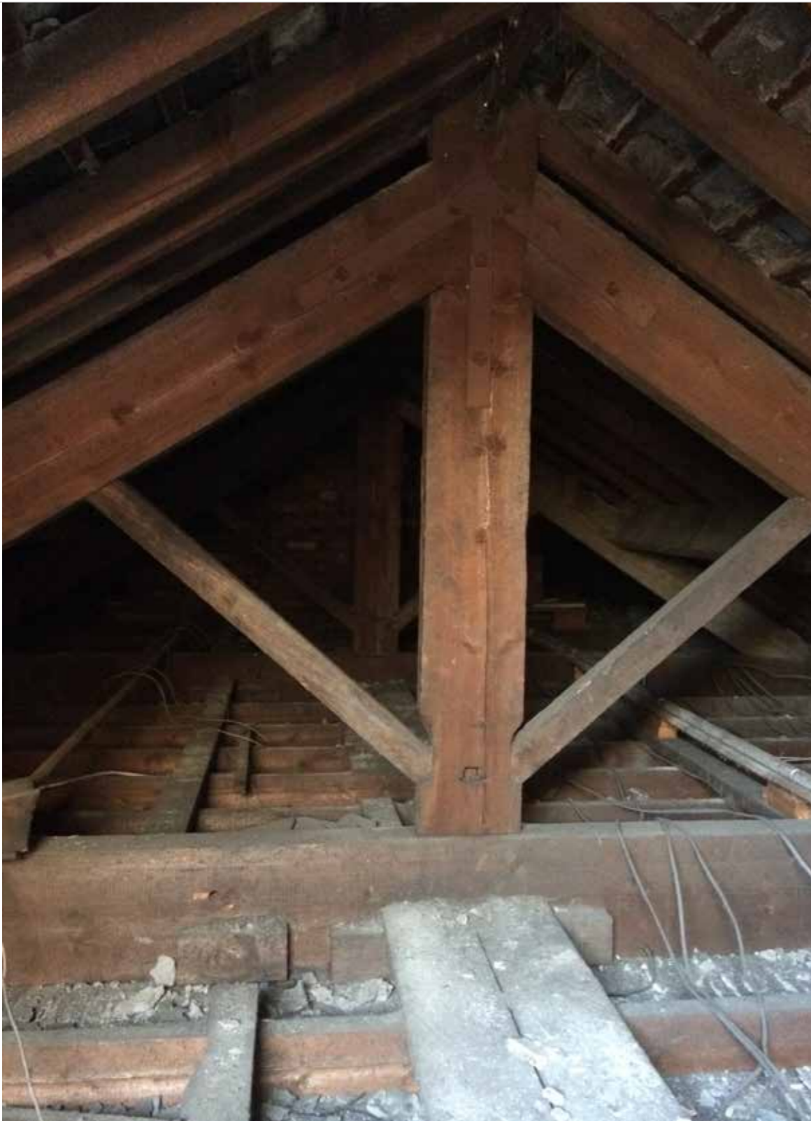
Existing Roof Structure
