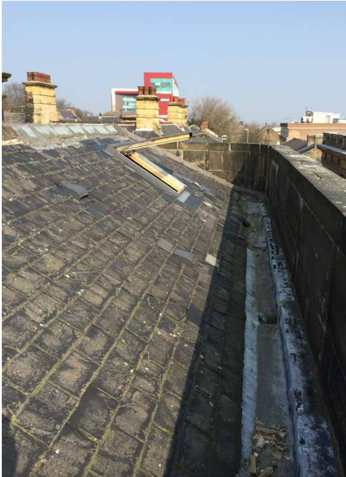
Existing Roof Looking North
