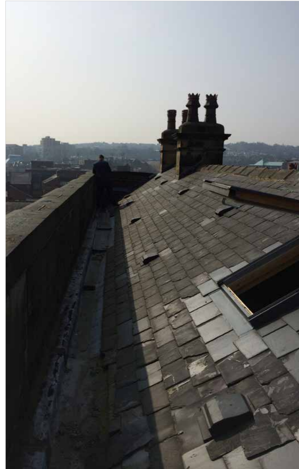
Existing Roof Looking South
