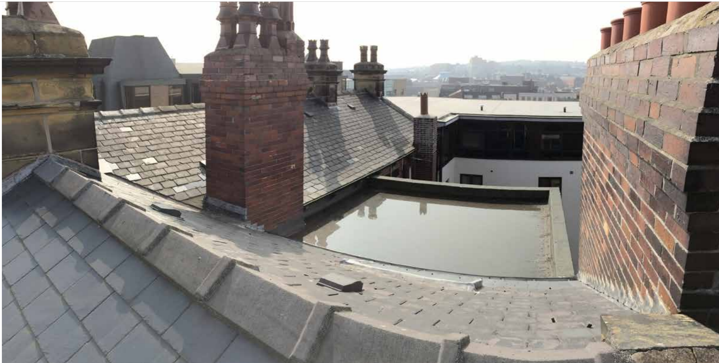
Existing Roof Looking into Courtyard
