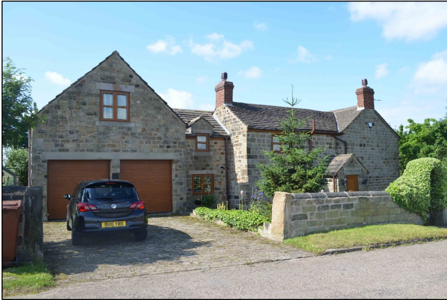
Figure 11: View of Woodbine Cottage, looking south
