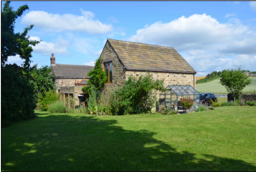
Figure 14: View of Woodbine Cottage, looking north-west
