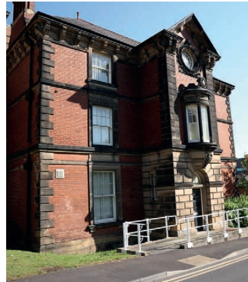
Above: 1862 former Beckett Hospital building to be retained and converted into 11 apartments
