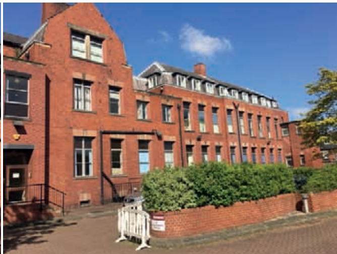
East elevation to be demolished
