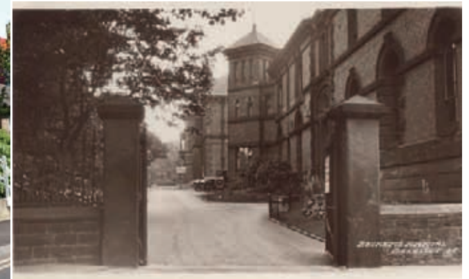
Above: Views of the larger Beckett Hospital site prior to demolition in the 1970’s
