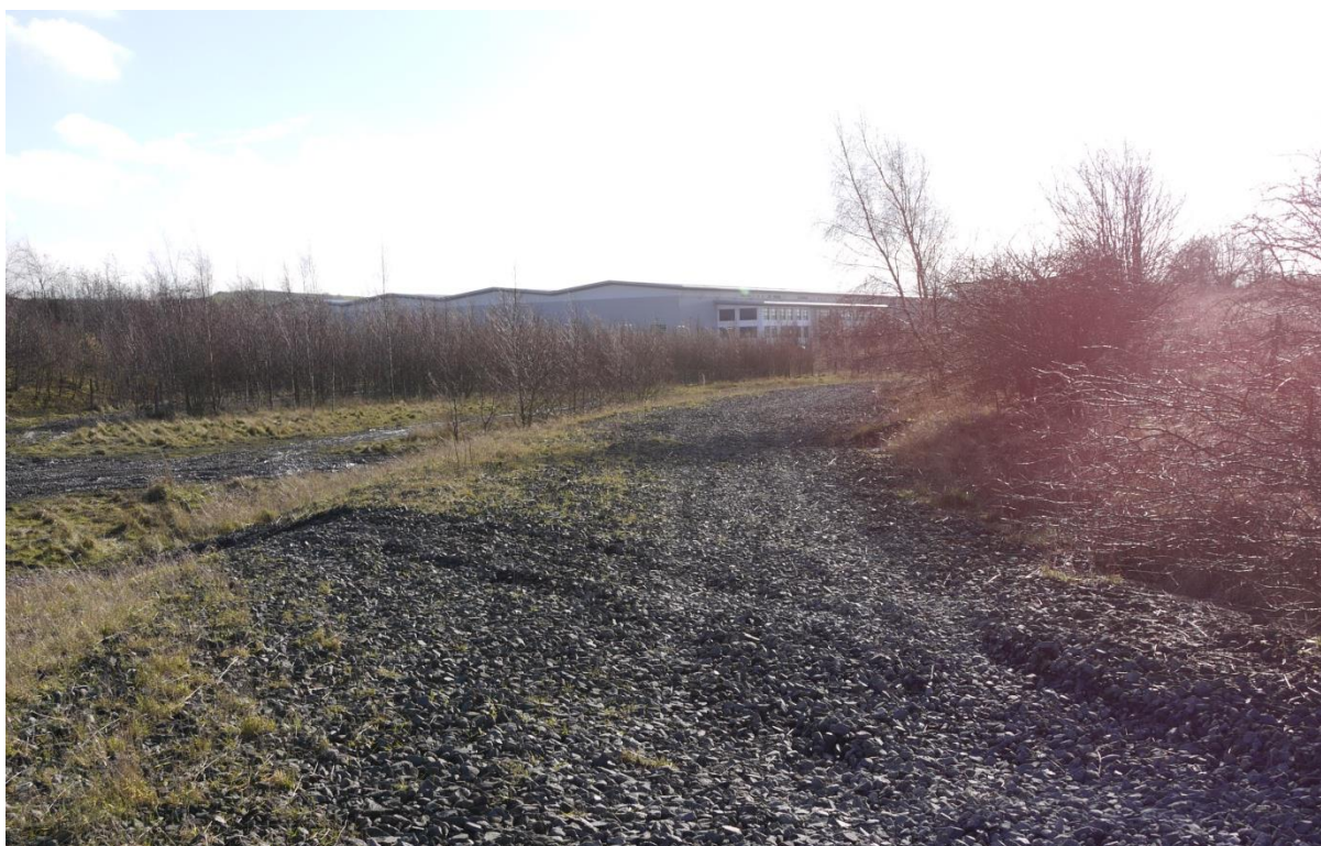
Photograph 3: View of the dismantled railway, forming the northern boundary.
