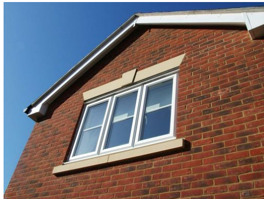
Plate 2.8 - Artificial stone cills and lintels
