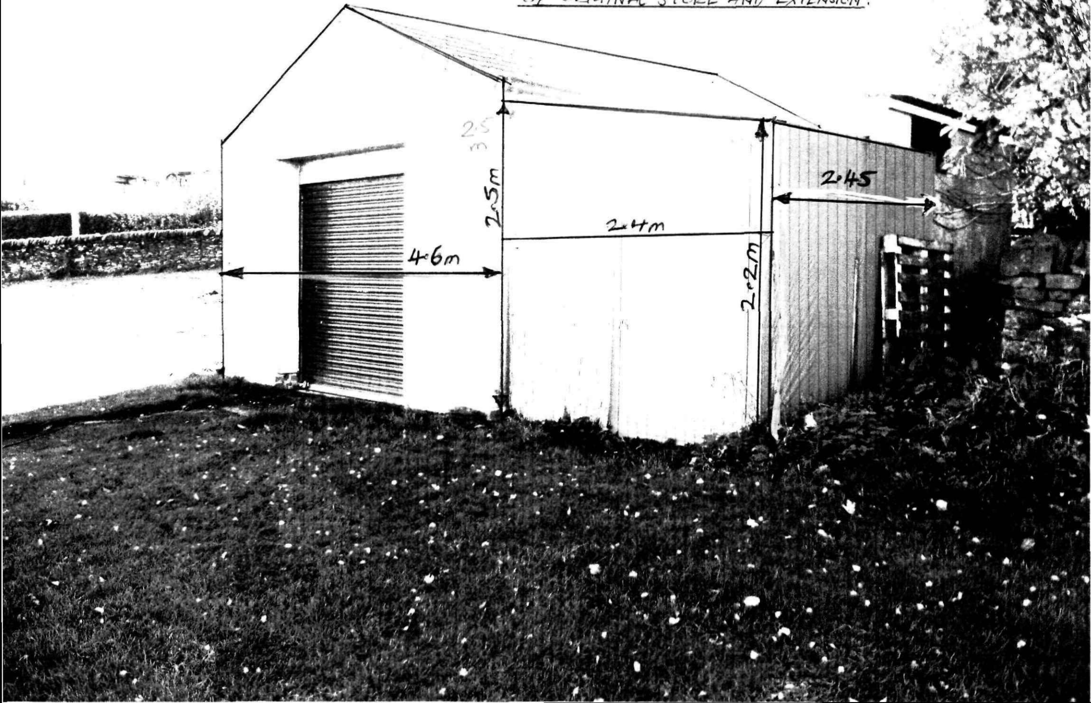
FIG 1 GENERAL PROPORTIONS OF ORIGINAL STORE AND EXTENSION.
