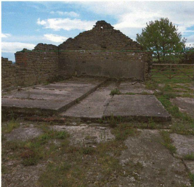
Photograph 2 – The Building Remains
